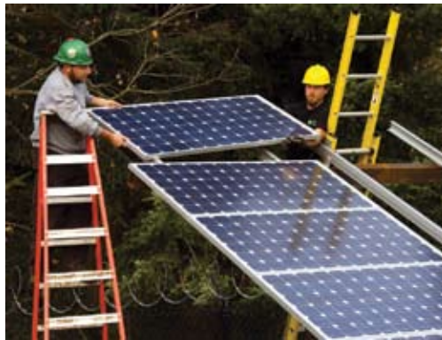
Solar energy installation jobs cannot be outsourced. Credit: Oregon DOT
